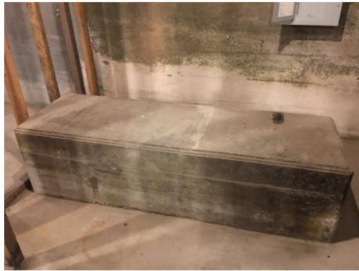
The cement box (casket) located in the basement of the old Hampden Academy brick building
